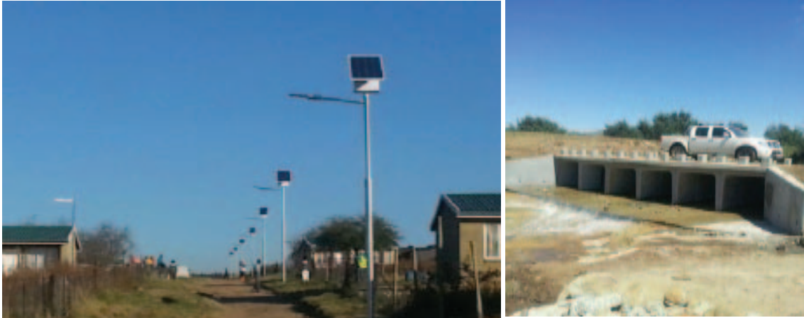
Jabulani houses and solar street lights and Donkerhoek low water bridge
