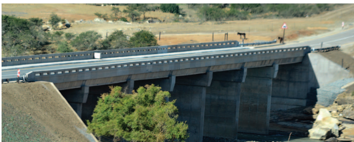
Nkosi Dalibunga Mandela Legacy Bridge and 10km access road
