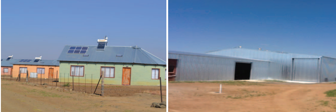
Diyatalawa solar water geysers and solar panels, Makholokoeng potato shed
