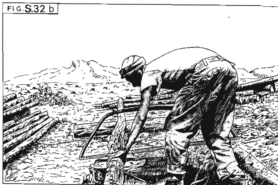
CROSSCUTTING POLES BY ONE-MAN BOW-SAW.
